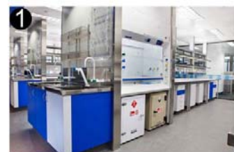
COMBINING FUME CUPBOARDS AND SINKS TO CENTRALISE SERVICES WITHIN THE PARTITION WALL
