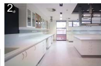
OVER HEAD STORAGE AND SERVICES ON THE WALL. DUCTS ALLOW TO LOCATE THE POWER SUPPLY WHERE NEEDED
